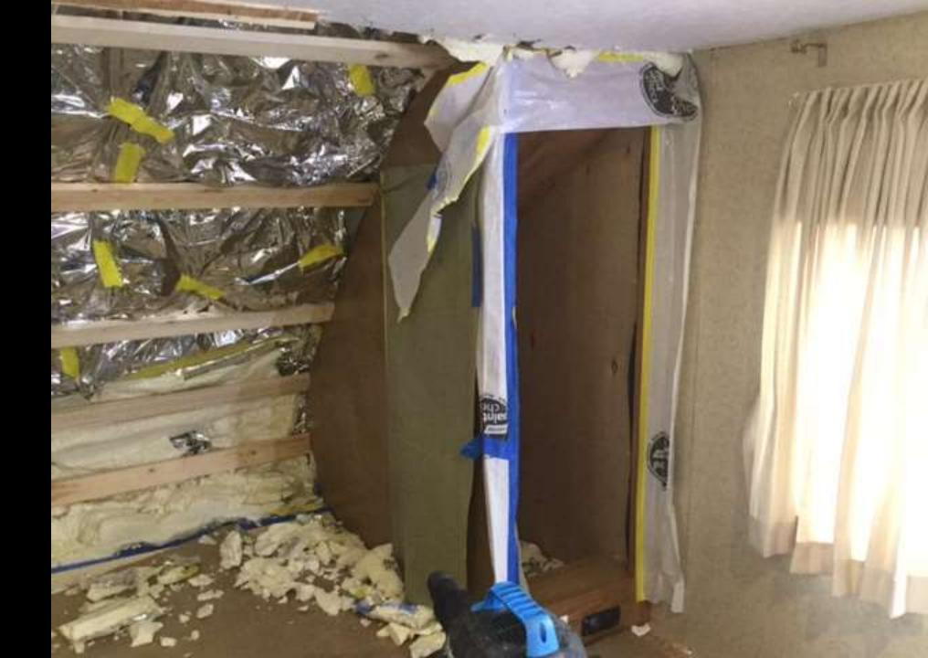
Closets reinforced to each other, screwed and glued to the trailer walls and frame. It's stronger and better insulated then it was from the factory for sure.
